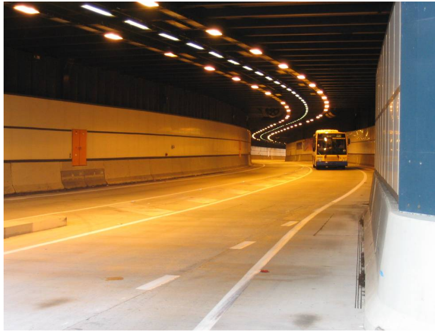
Photo 4.6 Brisbane South East Busway Tunnel
