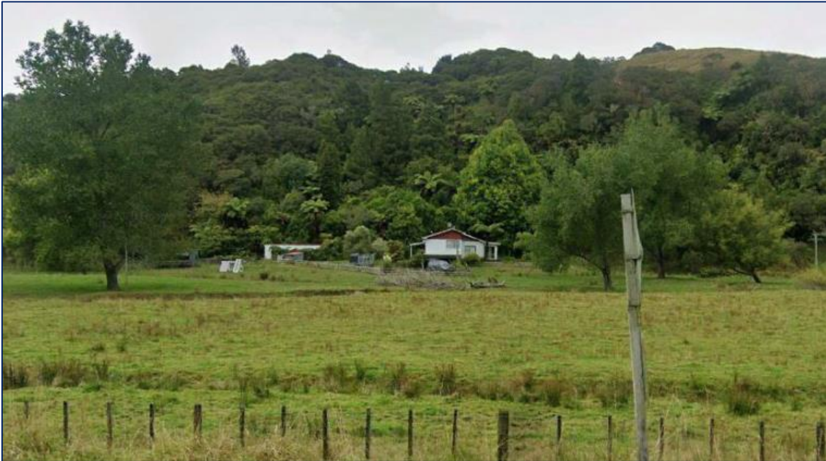
Figure 2: Street View of Dwelling at 2528 Mokau Road
