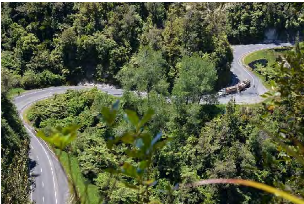
Photo 3.1 – SH3 at Mt Messenger viewed from the southern approach
