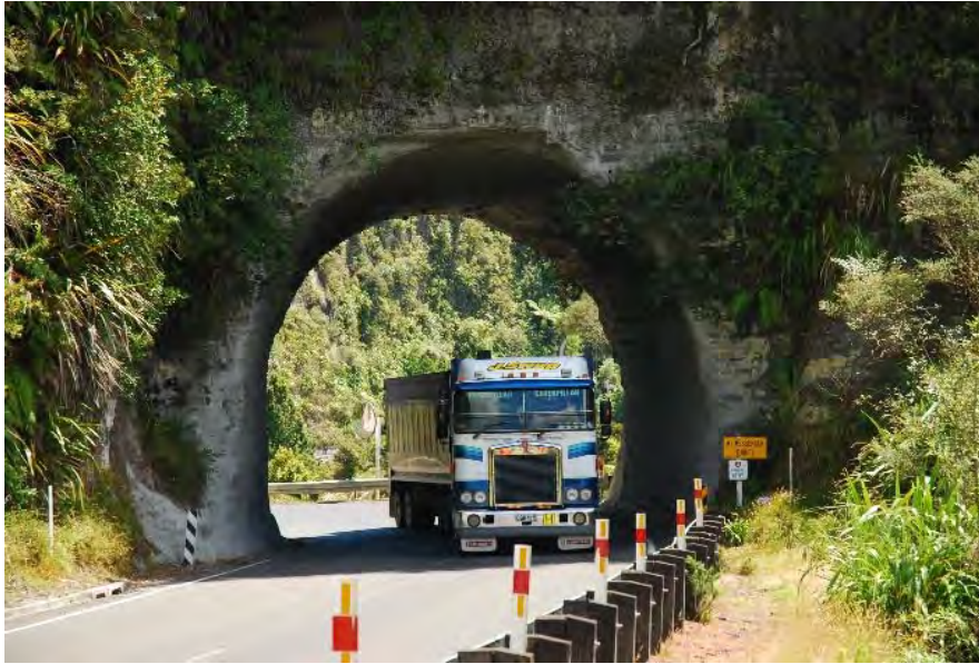
Photo 3.2 – Mt Messenger tunnel from the southern approach
