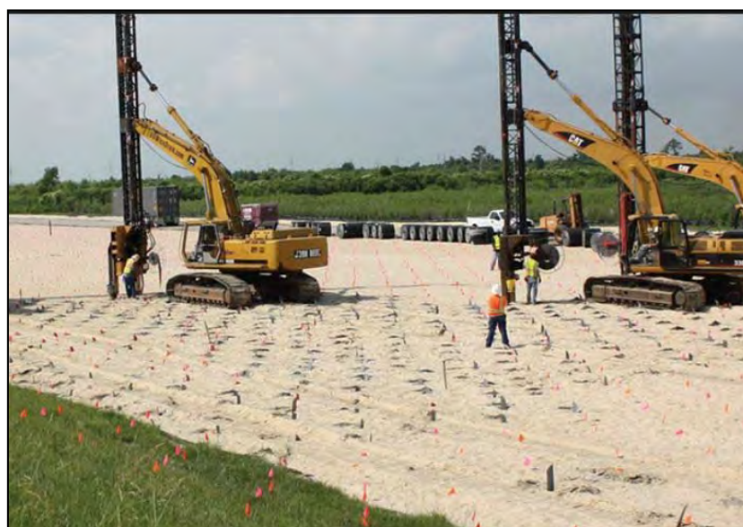
Figure 5.8 – Indicative wick drain layout
