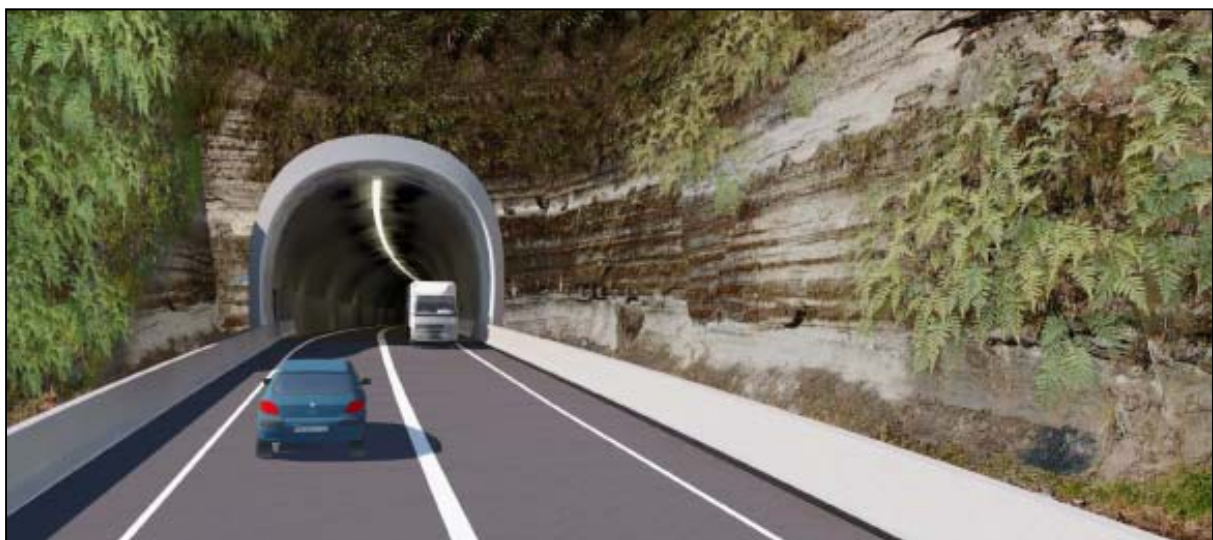
Figure 4.10 - Indicative view of tunnel approach showing the main tunnel portal and safety barriers
