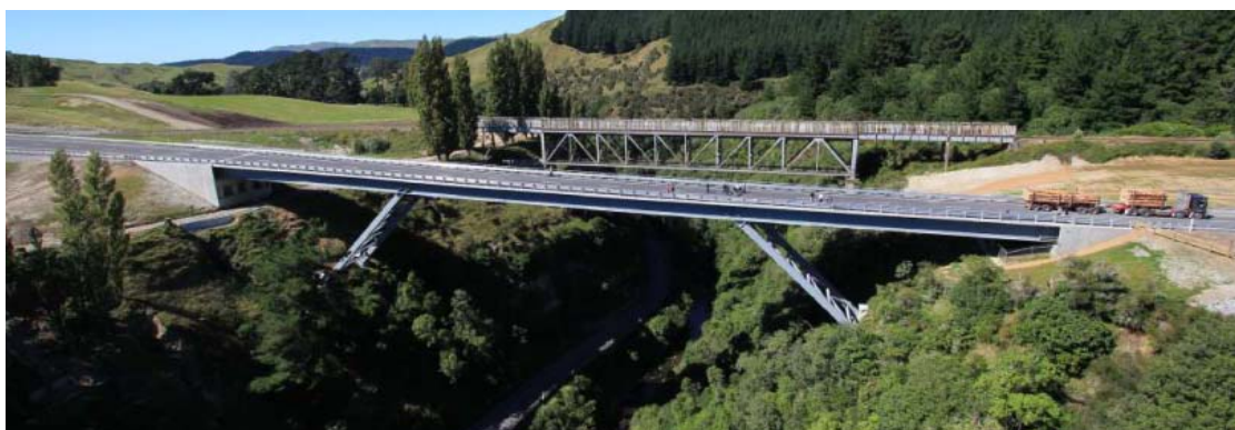
Figure 4.8 – Similar Bridge Arrangement (Matahorua Gorge)
