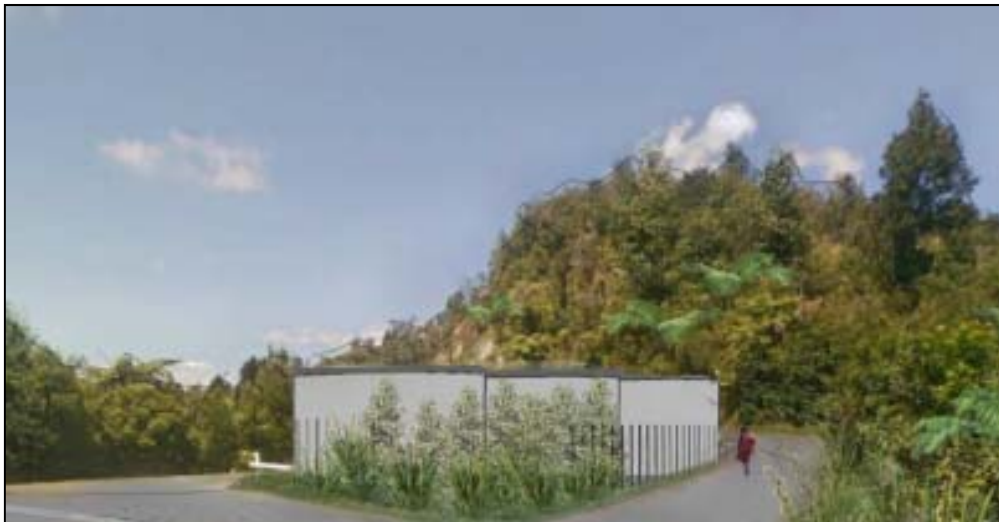
Figure 4.12 – Water tanks at the existing SH3 rest area
