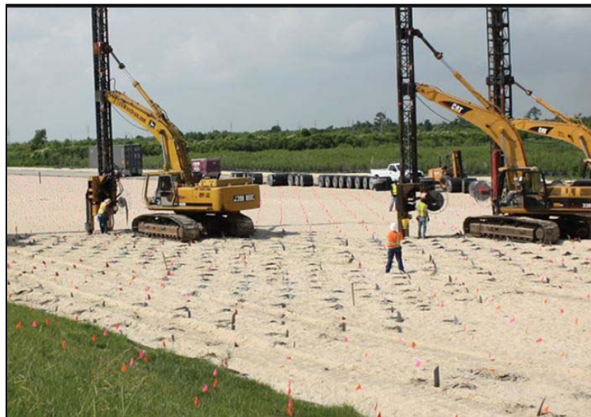
Figure 5.8 – Indicative wick drain layout
