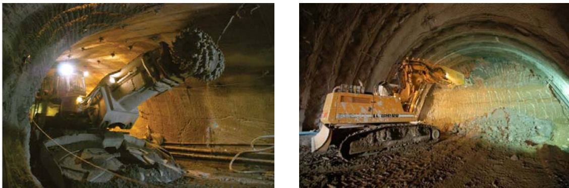
Figure 5.9 – Tunnel construction using a Roadheader
