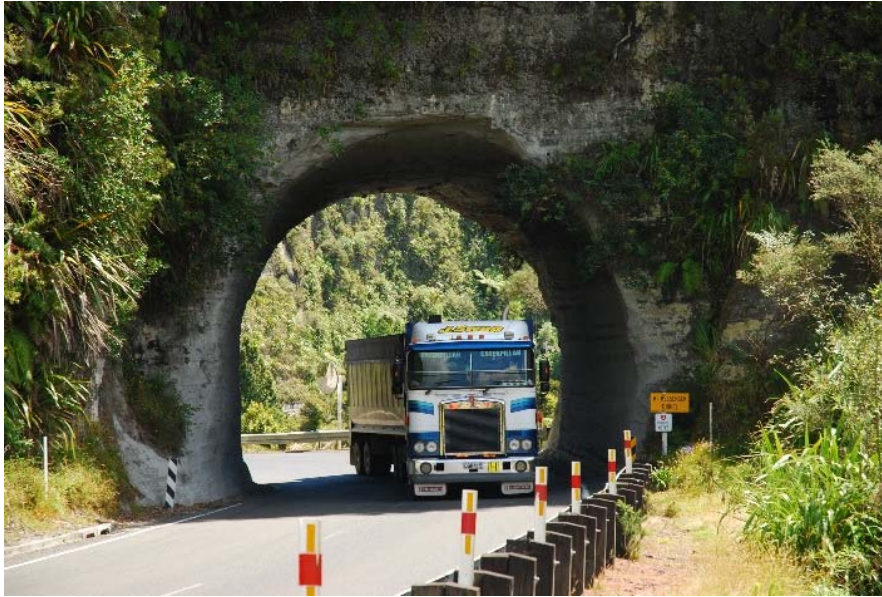
Photo 3.2 – Mt Messenger tunnel from the southern approach
