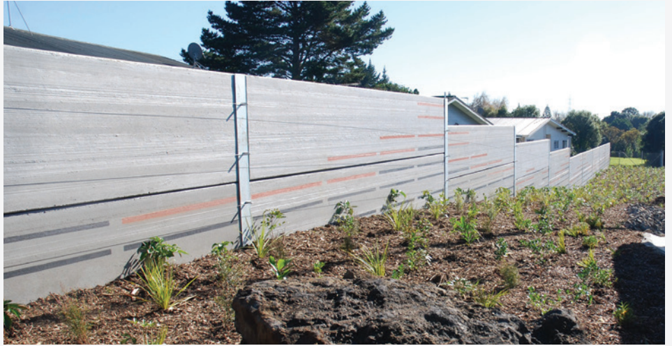
Existing noise wall Takanini – Using concrete panels between steel posts
