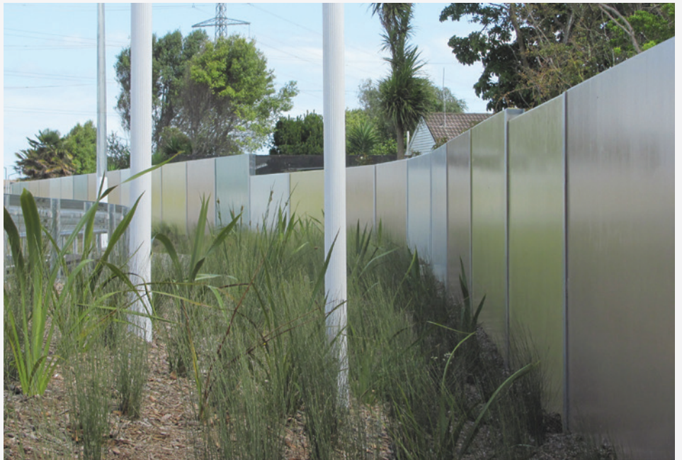
Existing noise wall Papakura – The palette was selected to reference the landuse and environment, along the route of the wall. Therefore, it has more green and blue paint tones towards the coast and moves into more earth tones (greens and browns) towards Papakura where there was a long history of agriculture and horticulture.
