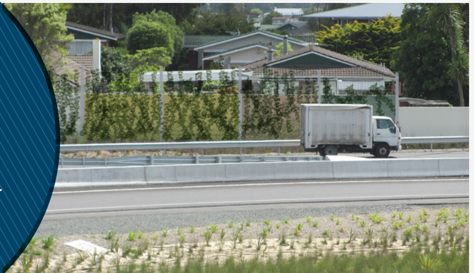
In the Conifer Grove area it's proposed that a vertical extension to the noise barrier in this location will support plant growth i.e. climbers to reflect the green in the area at present. *Artist impression only.
