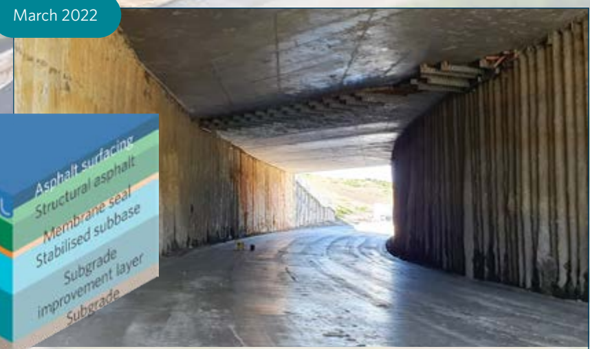
Below SH1 the 120m long underpass provides a seamless connection for people and goods travelling from the north and heading west which will help make journey times around the region more reliable. To build the road itself, many layers like those of a cake are required to ensure it has the necessary strength and durability. Work on the first layer started in March this year.
