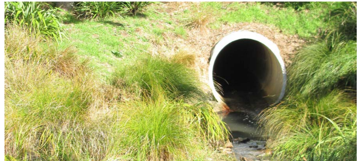
Culverts chamfered to be recessive and naturalised watercourse
