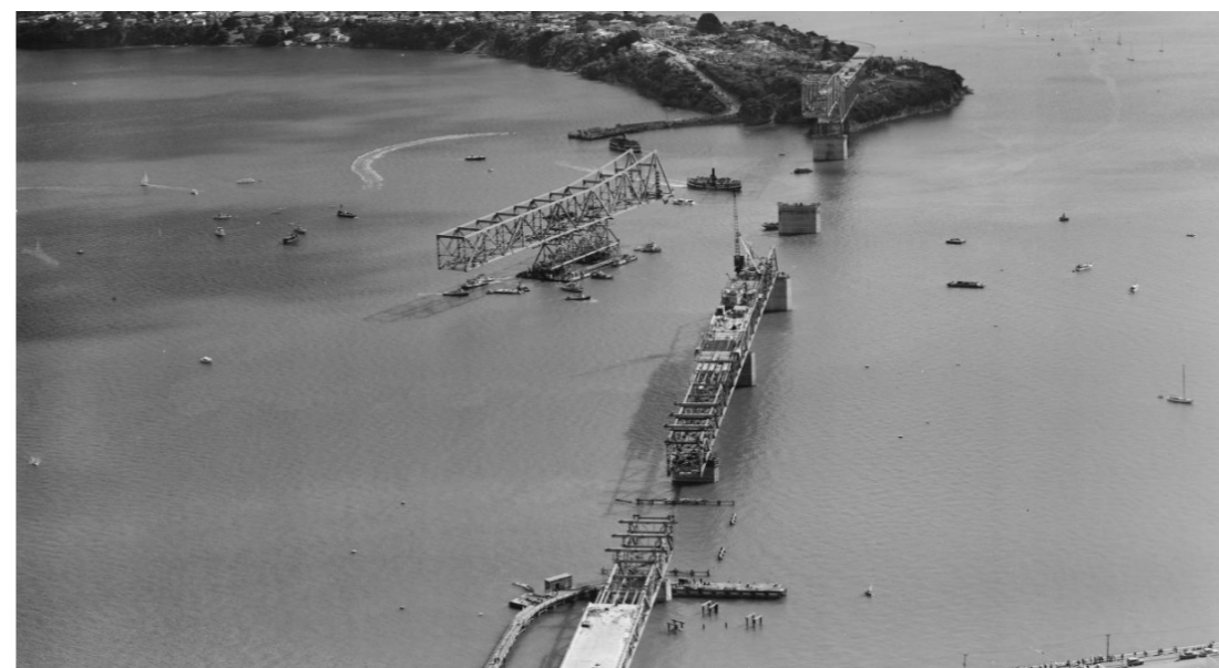
Auckland Harbour Bridge under construction Source: Auckland Motorways, NZ Transport Agency 2008
