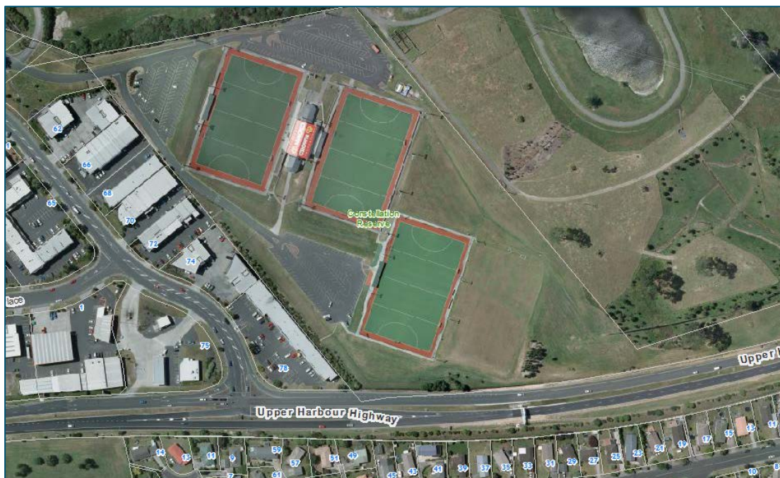
Figure 7 Aerial image of North Harbour Hockey Stadium
