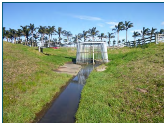
Figure 25 Stormwater Drain Discharge Point Through Vertical Culvert
