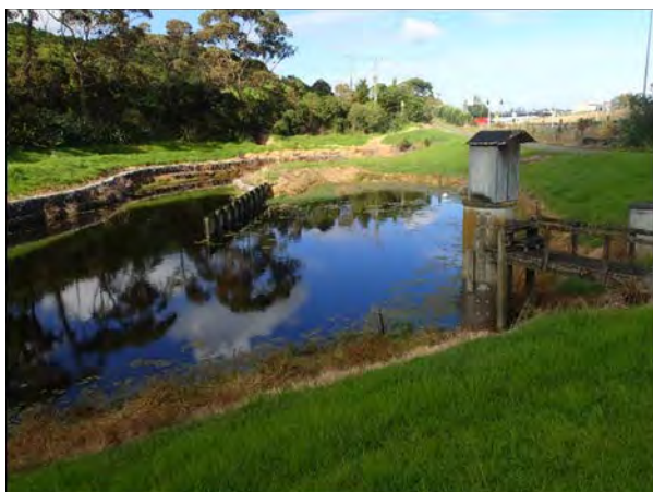
Figure 19 SWP 7 Rosedale Closed Landfill
