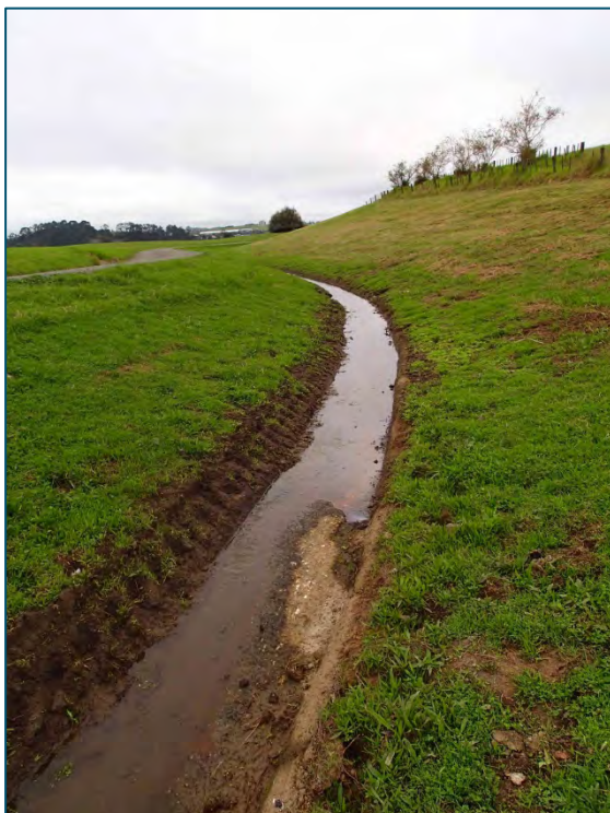
Figure 37 Stormwater Drain adjacent to Pond 1
