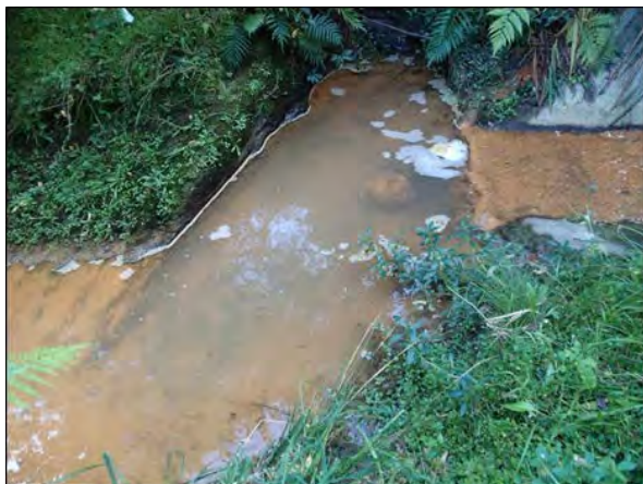
Note: Culvert apron on right and discharge pool
