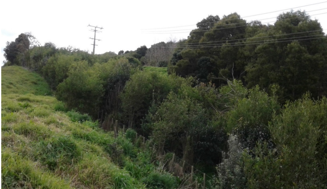
Figure 7 Rosedale Landfill – a rough hedge has become established on the boundary consisting of Tasmanian Blackwood ( Racosperma melanoxylon ) and other pioneer species such as Kohuhu. There is a relatively level strip of ground along the top of the existing motorway cutting, which can be seen at left
