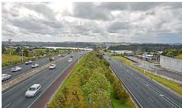
Construction of the Northern Busway Extension will be complete by 2021.
