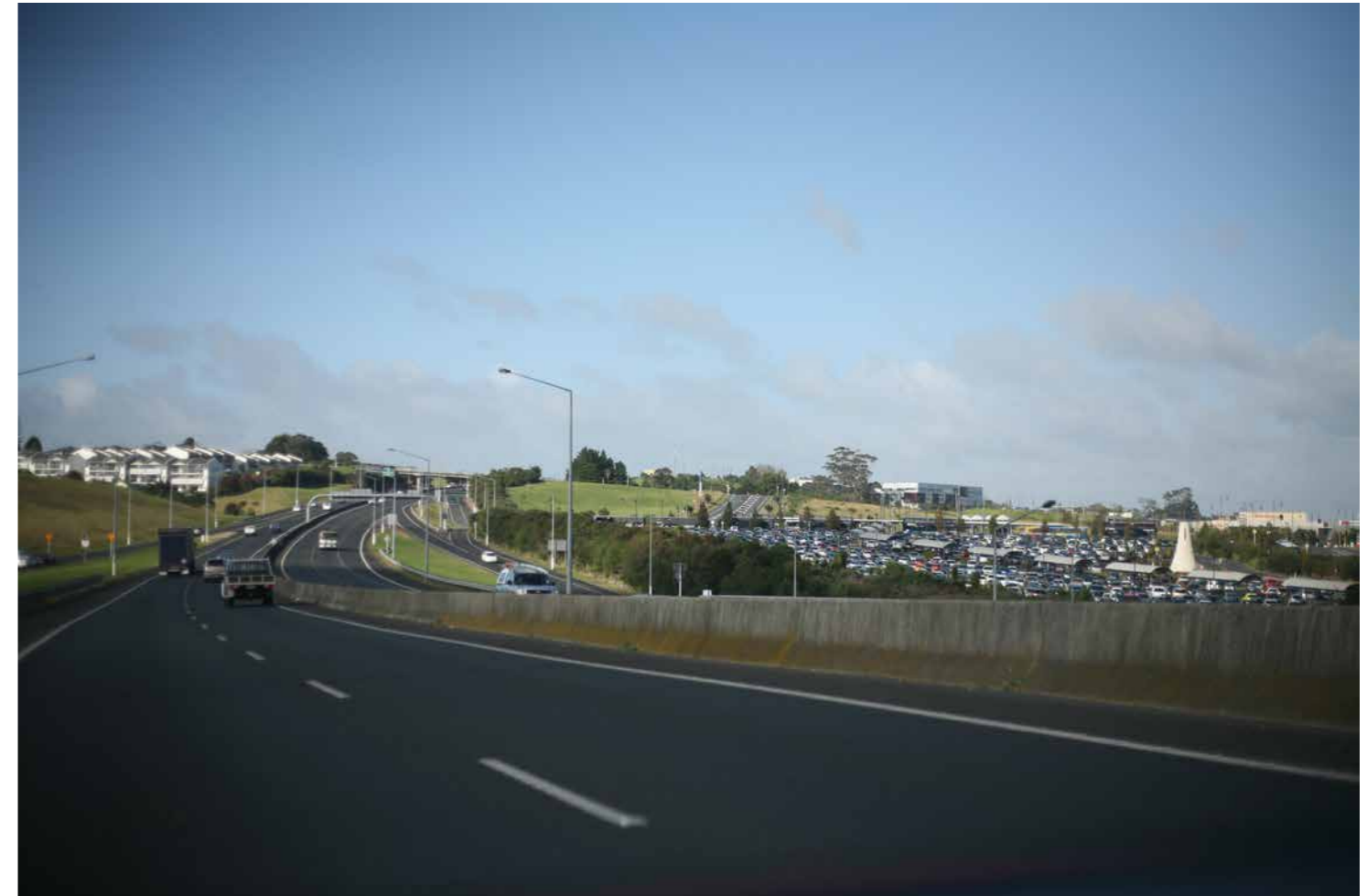
Viewpoint D: Southbound over Oteha Valley Road
