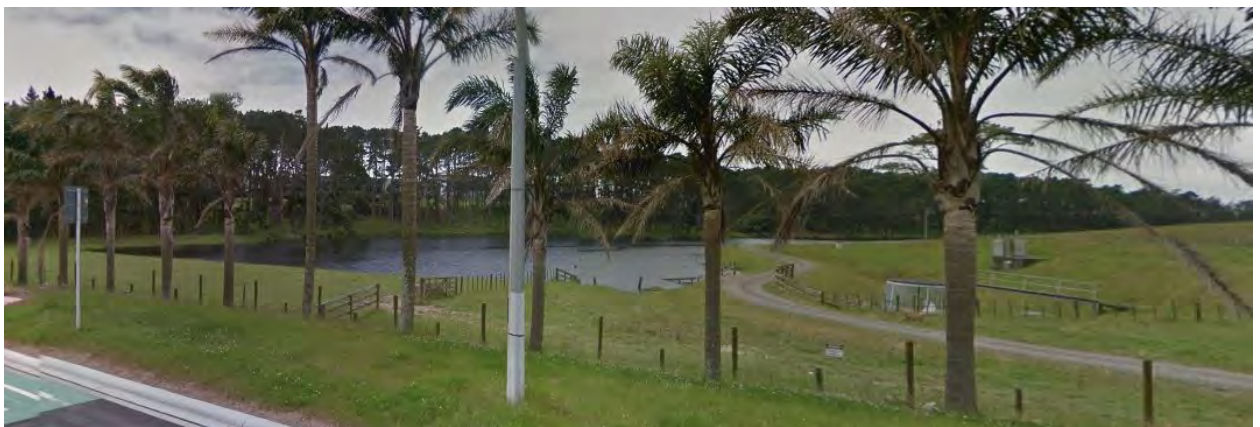
Fig 5.5 Ti Kouka Rosedale WWTP southbound
