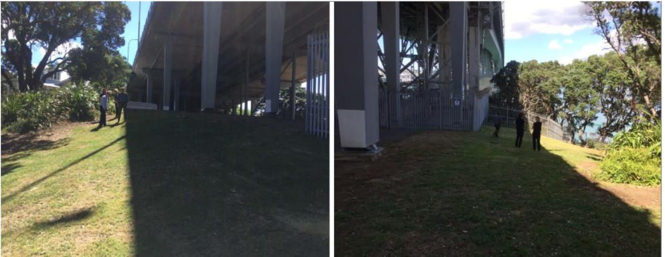
2 February 2021. Western Park; LHS – view to north towards #1 Queen Street from North Anchorage; RHS – view to south showing North Anchorage.
