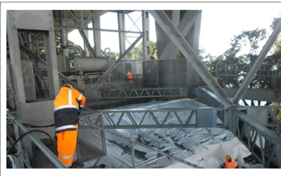
Figure 2.2: Containment system over Stokes Point to collect wet abrasive blasting wastewater
