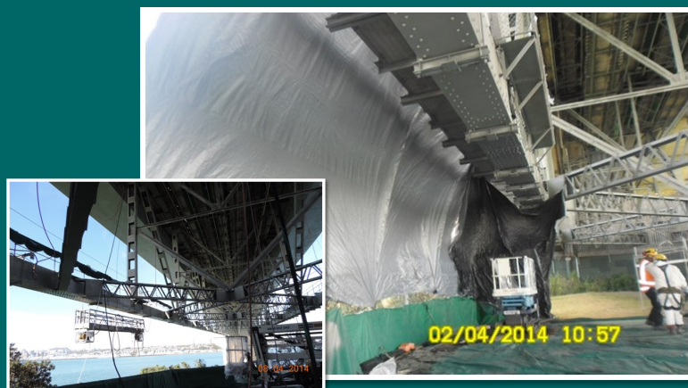
Figure-1 Containment at Stokes Point Reserve
