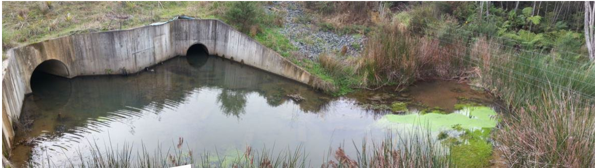
Photo 2 - Riprap basin for NGTR Nukumea culverts.
