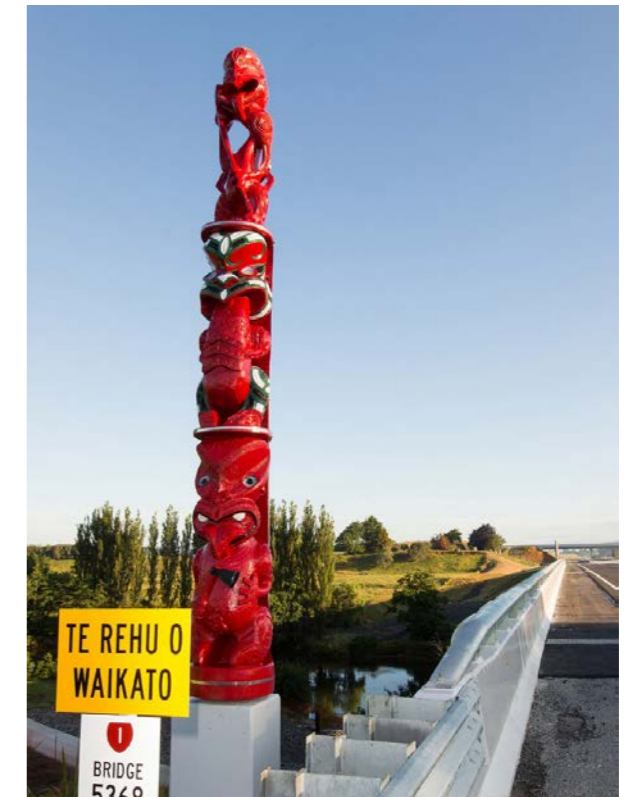
Waikato expressway pou at Waikato River Bridge
