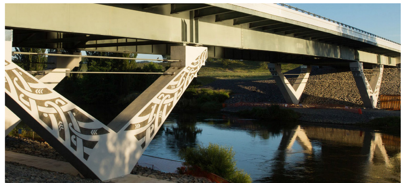
Art integrated to Waikato River bridge. Bridge form completely outside the river bed.
