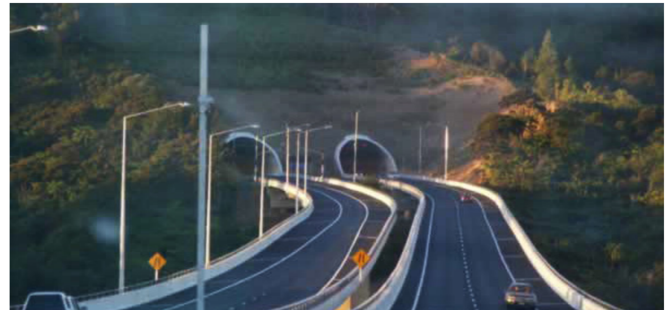
Johnstones Hill Tunnels are a good example of tunnel portal integration with the landscape. The portals were extended beyond the tunnel and truncated at a similar angle to the adjacent landform.
