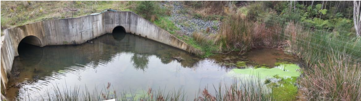
Photo 2 – Riprap basin for NGTR Nukumea culverts.
