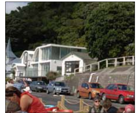
As Built View
