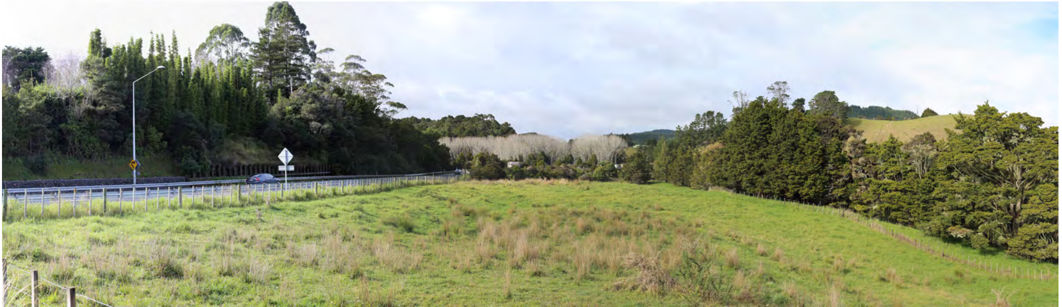
Viewpoint 8: SH1 looking south-east
