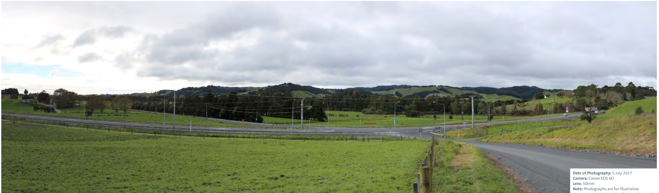
Viewpoint 9: Wayby Station Road looking east
