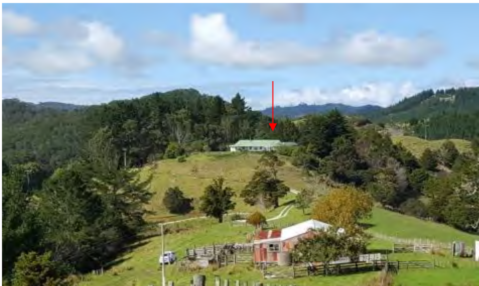
Figure 68 – Modern house built near the southern extent of the property at 1207 SH1 (red arrow).
