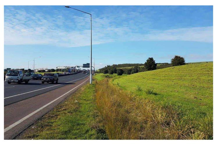
The design, construction and operation of state highways can potentially affect natural waterways and drainage patterns. Although careful consideration is taken during design and route selection, the alignment of some state highways can intercept waterways and overland flow paths, increase erosion rates and potentially increase flood flows.
