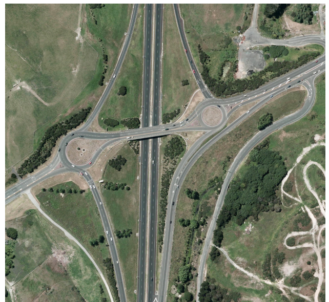
Silverdale interchange showing ramps connecting to local roads
