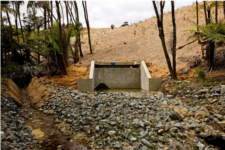
Figure 10 - Diversion of stream flows around the culvert work area
