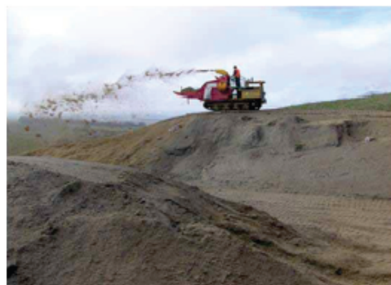
Erosion Control – Mulching
