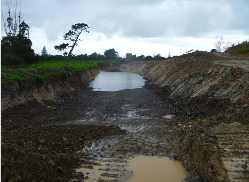
Figure 12 – Shear Key excavation
