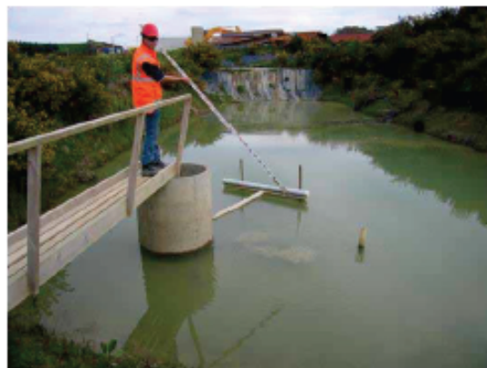
Undertaking Maintenance of a Sediment Retention Pond
