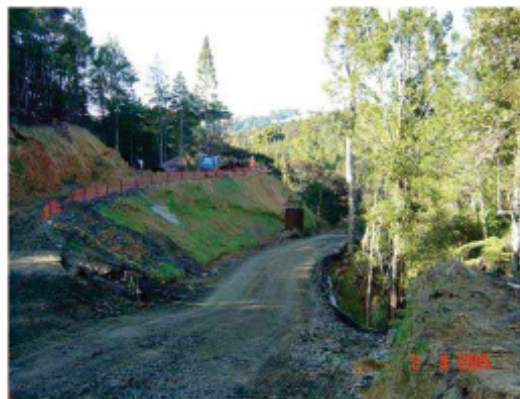
Highway Construction Site – Minimising Disturbance
