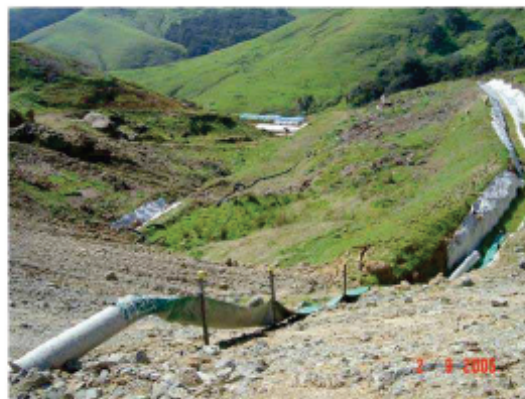
Flume Installed to Protect Steep Slope
