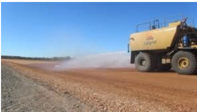
Figure 15 - Water cart dust suppression
