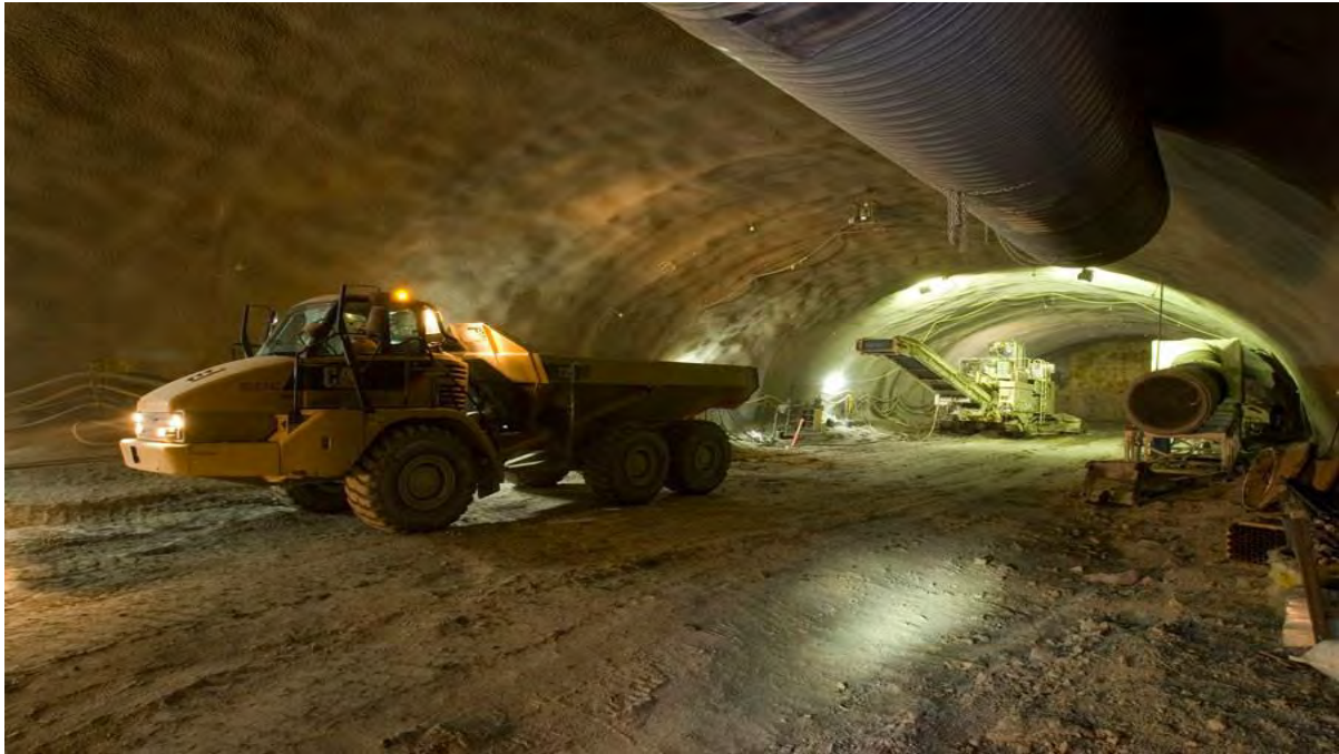
Figure 5-8: Excavation of lower bench by rock milling machine
