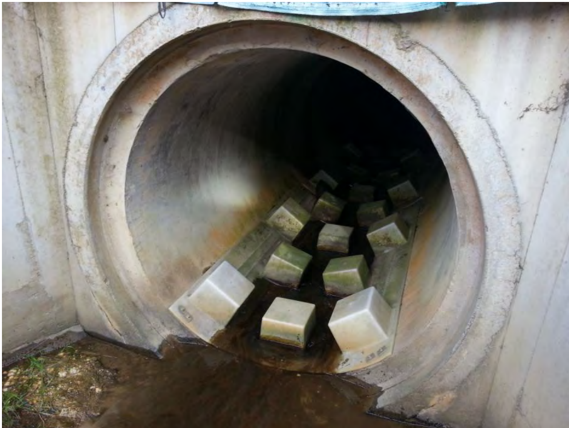
Figure 4–8: Baffle type fish passage installed at Waiwera
