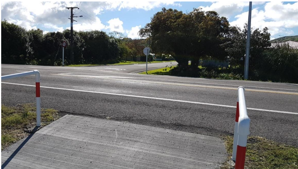
Figure 6: Lateral shared path connections at Murdoch Road
