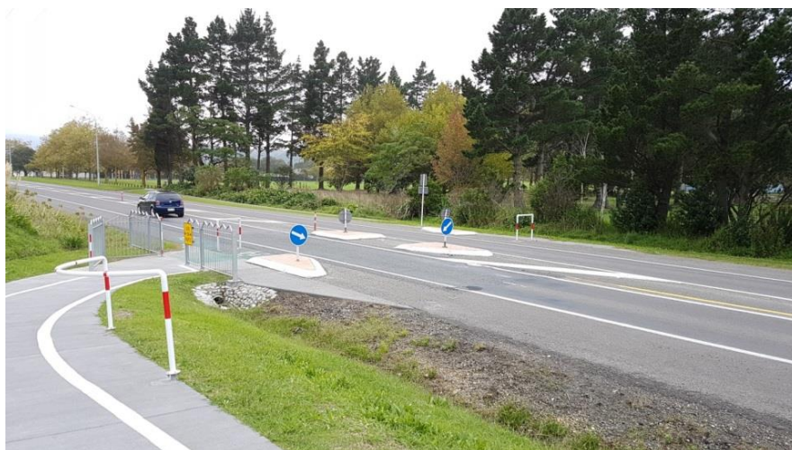
Figure 2: Termination of shared path at 70 kph zone.
