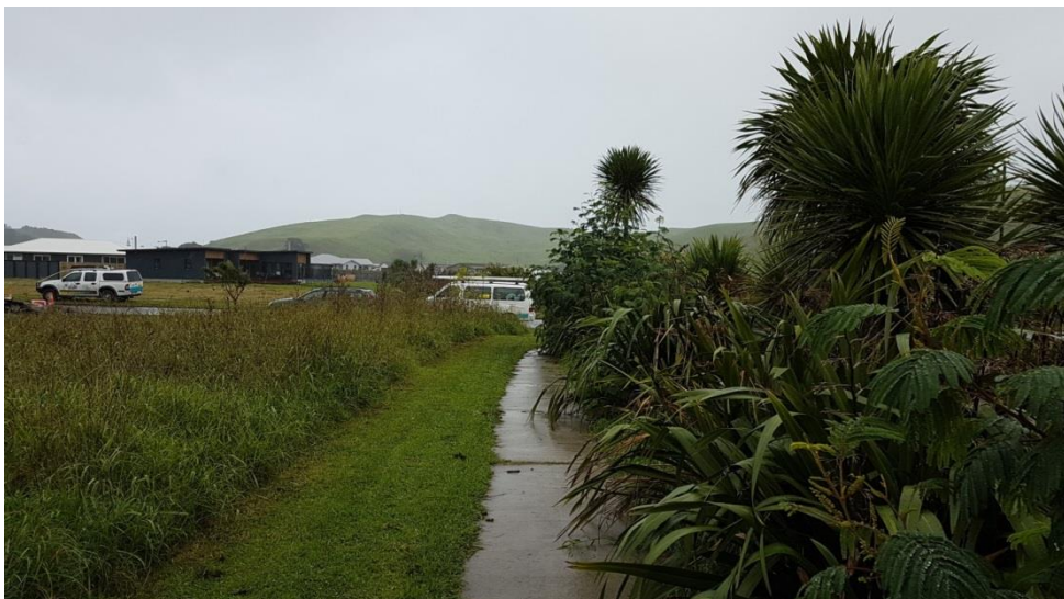
Figure 8: Encroaching vegetation on access way
