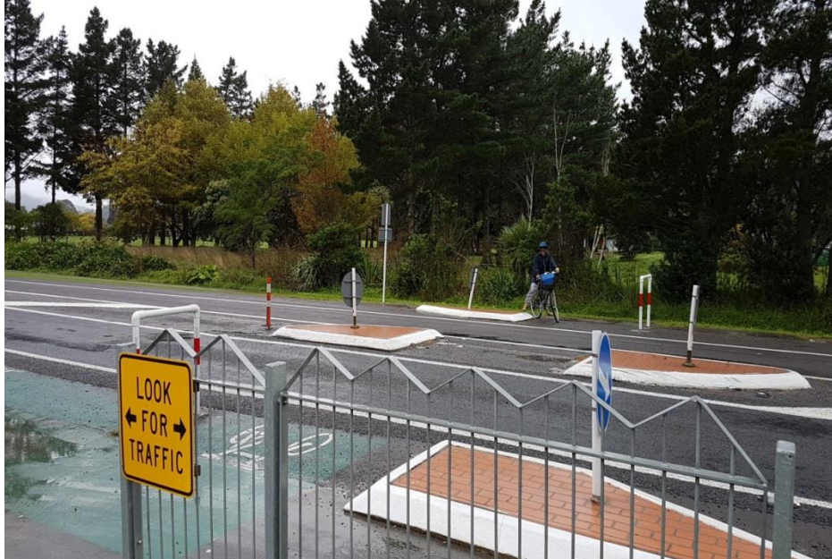
Figure 13: Steel safety railings
