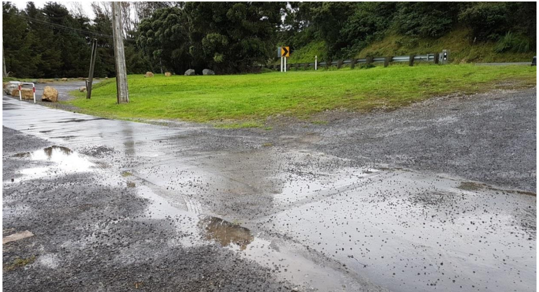
Figure 11: Significant chip loss on Wainui Road
