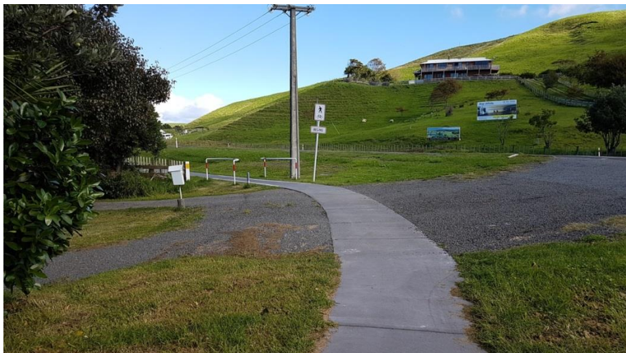
Figure 12 : Section of shared path below minimum widths
