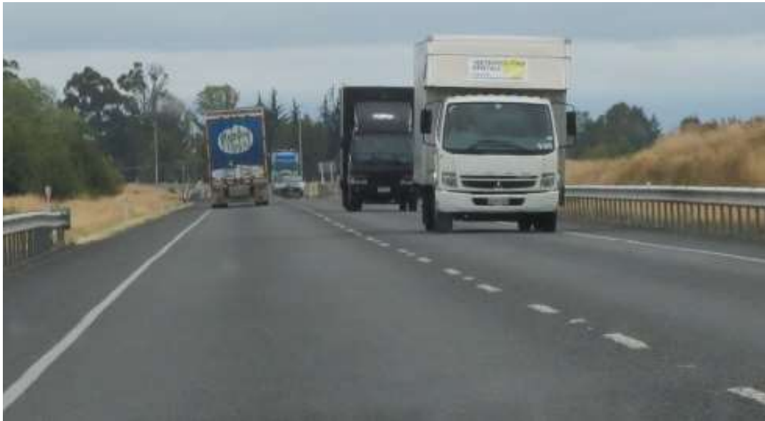
Figure 6: Trucks heavily use the bypass, diverting them from Taupo township
