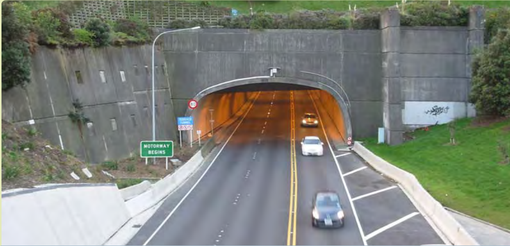
The southern portal entrance to the Terrace Tunnel. Completed in 1977, it was originally designed to have a twin. The Road of National Significance will realise the original plan.
