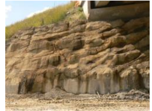
Artificial Rock Bridge Abutment
