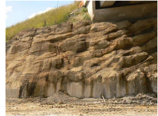
Artificial Rock Bridge Abutment
