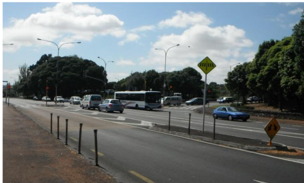
St Lukes Bridge Interchange
