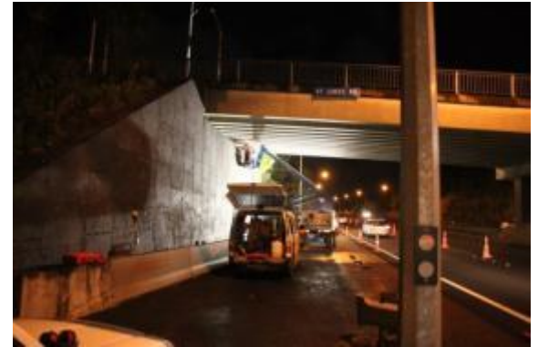
St Lukes Bridge Abutment
