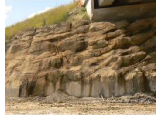
Artificial Rock Bridge Abutment
