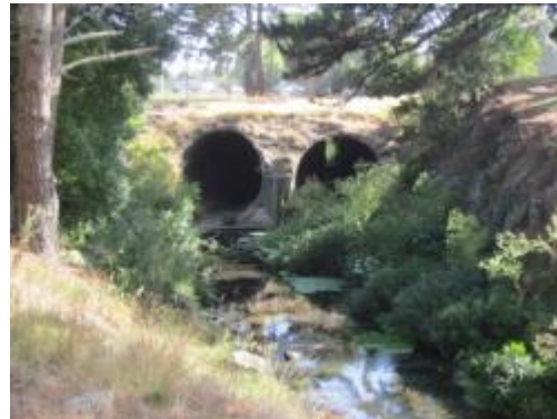
Meola Creek Culverts
