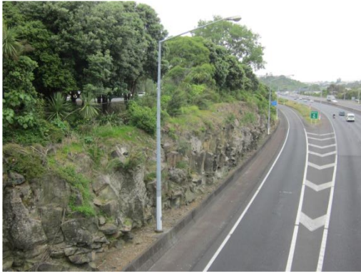
Basalt at St Lukes EB off ramp
