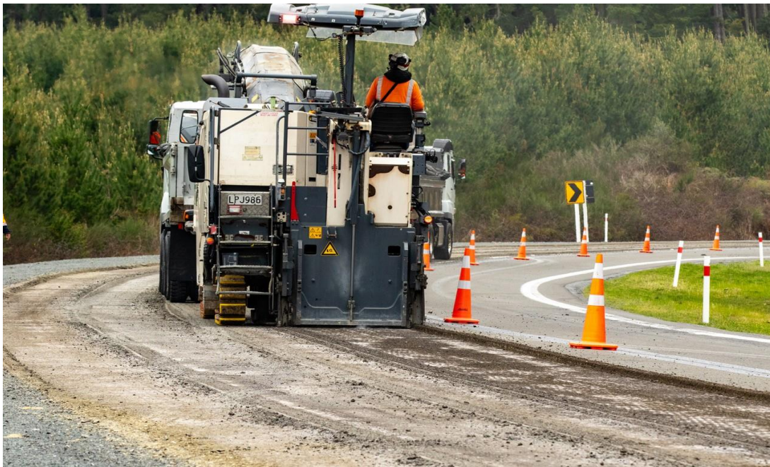
SH1 Wairakei – milling machine in action
