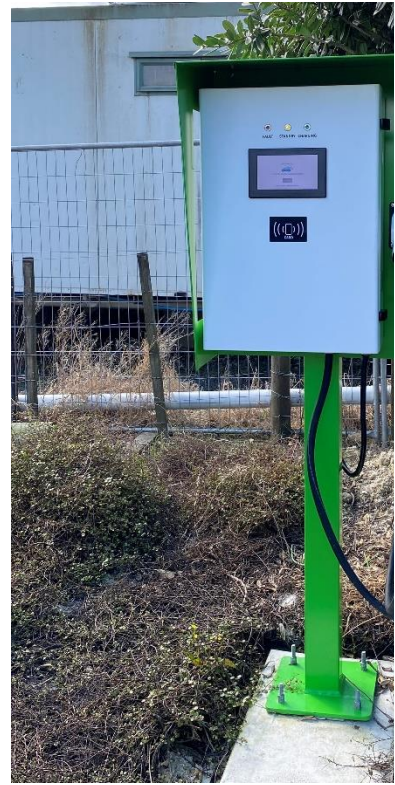
Close up of new charger installation
