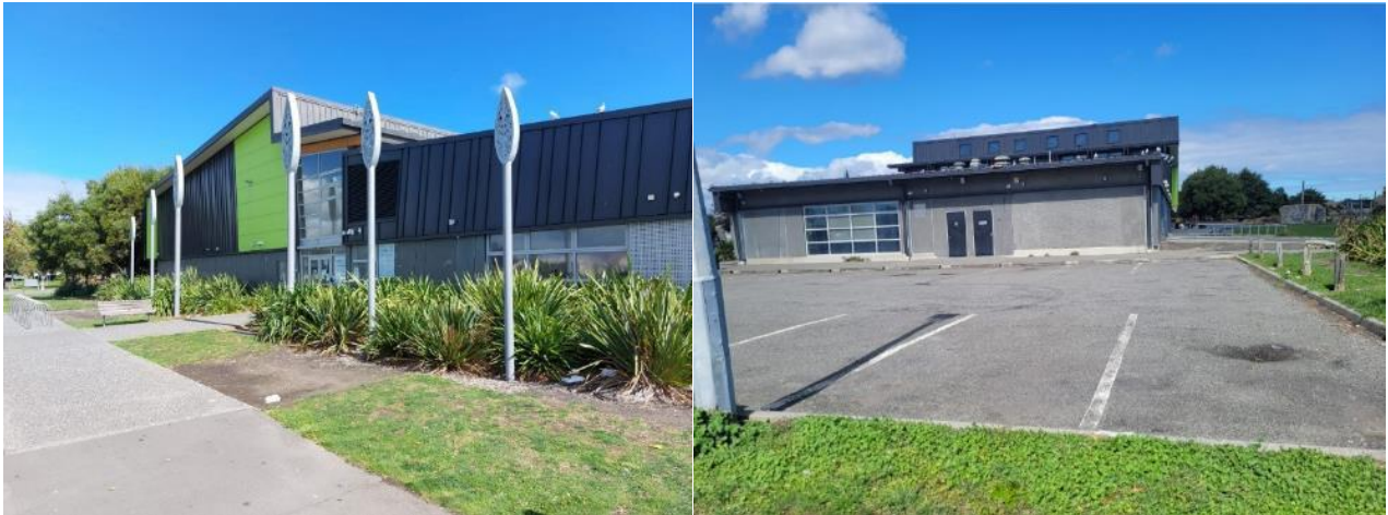
Figure 8.3: Wainoni Community Centre Entrance and bike stands (left), Wainoni Community Centre Northern car park (right)
