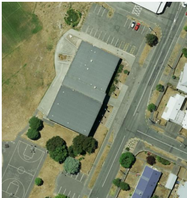
Figure 9.1: Wainoni Community Centre Aerial View of Northern and Southern Carparks
