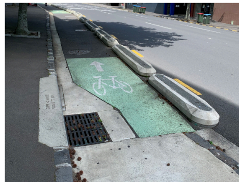
Typical drain causing hazard to trikes and sharp turn from footpath
