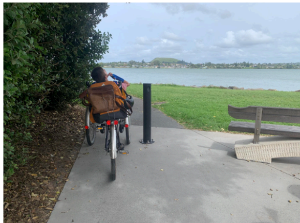
This post is at the Farm Cove public toilets. The only side we can access is just 1m in width. For cycling, this acts as a pinch point to navigate.
