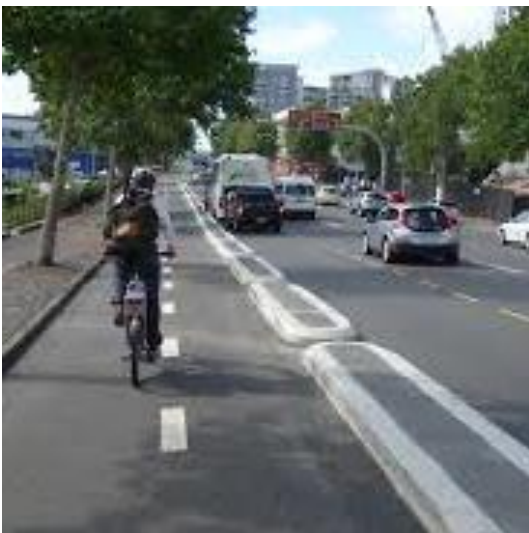
Figure 3A. A separated lane with small concrete barriers.
