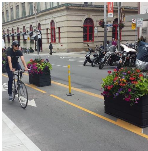
Figure 3B. A separated lane with planters.
