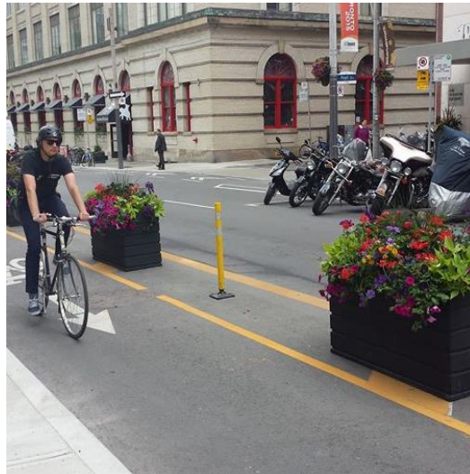
Figure 3B. A separated lane with planters.
