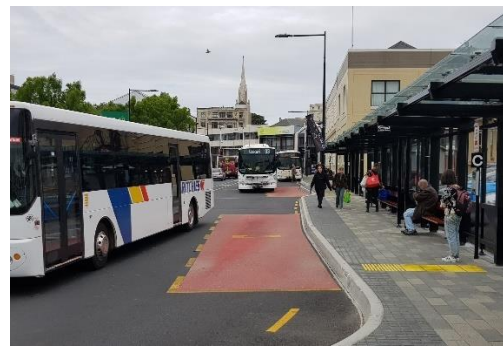
Figure 67: Shallow sawtooth or forward-exit sawtooth DIDO at Dunedin interchange. Source: Glen Koorey.
