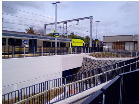
Figure 25: Pedestrian underpass, Tretham Station. Source: YttriumShrew, CC BY-SA 4.0, https://creativecommons.org/licenses/by-sa/4.0/ , via Wikimedia Commons
