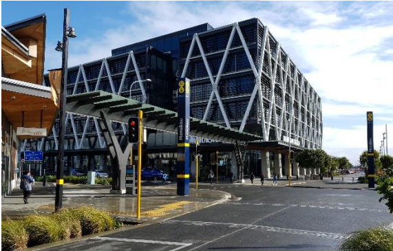
Figure 43: Manukau Station rain protection does not match desire lines and obscures the train station name. Source: Duncan Rothwell
