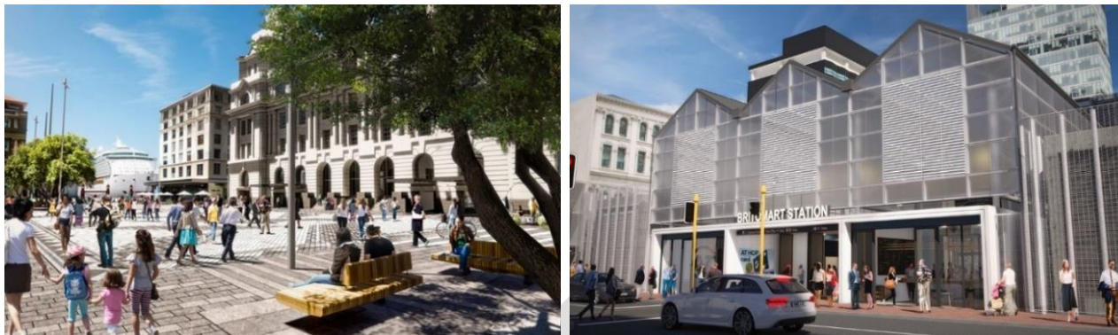
Figure 76: Britomart Transport Centre. Source: Auckland Transport.
