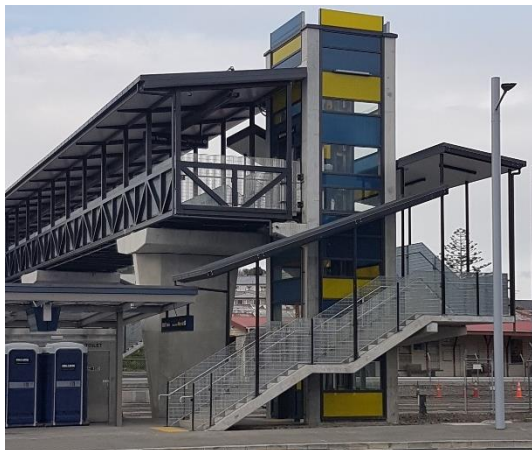
Figure 24: Pedestrian overbridge, Akoranga Station. Source: Auckland Council.
