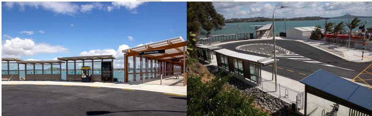
Figure 97: Half Moon Bay ferry pier and bus interchange. Sources: Auckland Council.
