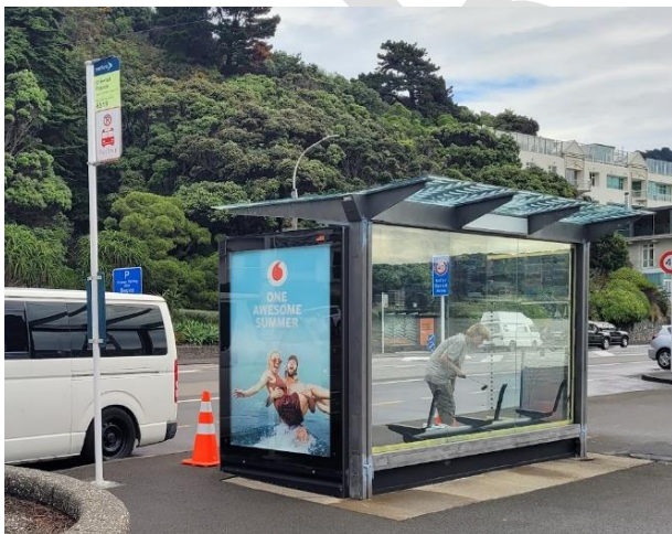
Figure 75: Bus shelter maintenance. Source: Lorelei Schmitt.
