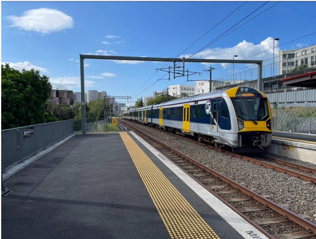
Figure 74: Train stabling area. Source: Jacobs.
