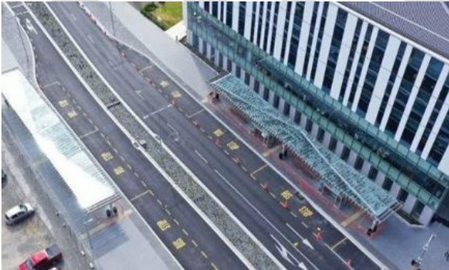
Figure 91: Christchurch Hospital bus stops. Source: Christchurch City Council Newline.
