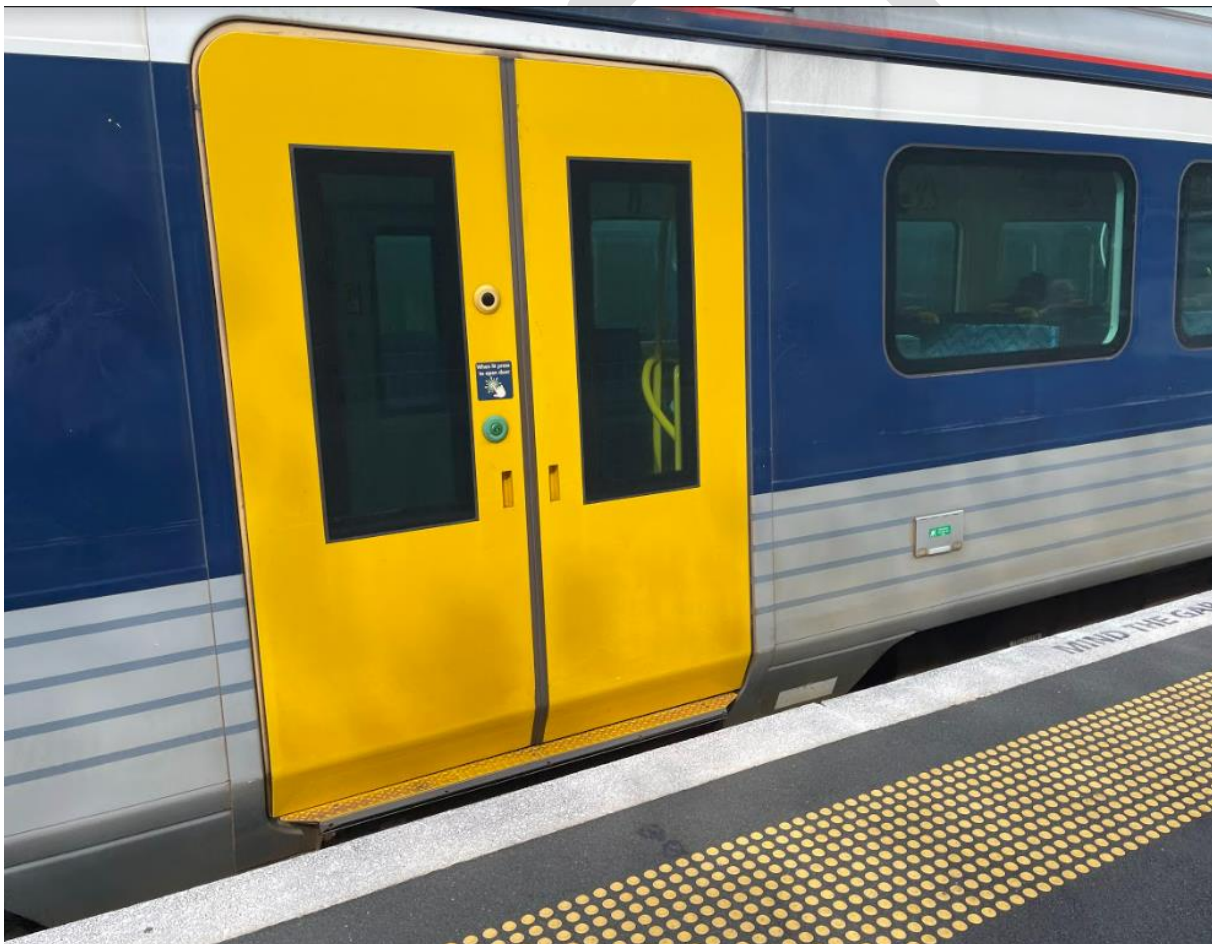
Figure 29: Tactile ground surface indicators along the length of a train platform. Source: Jacobs.
