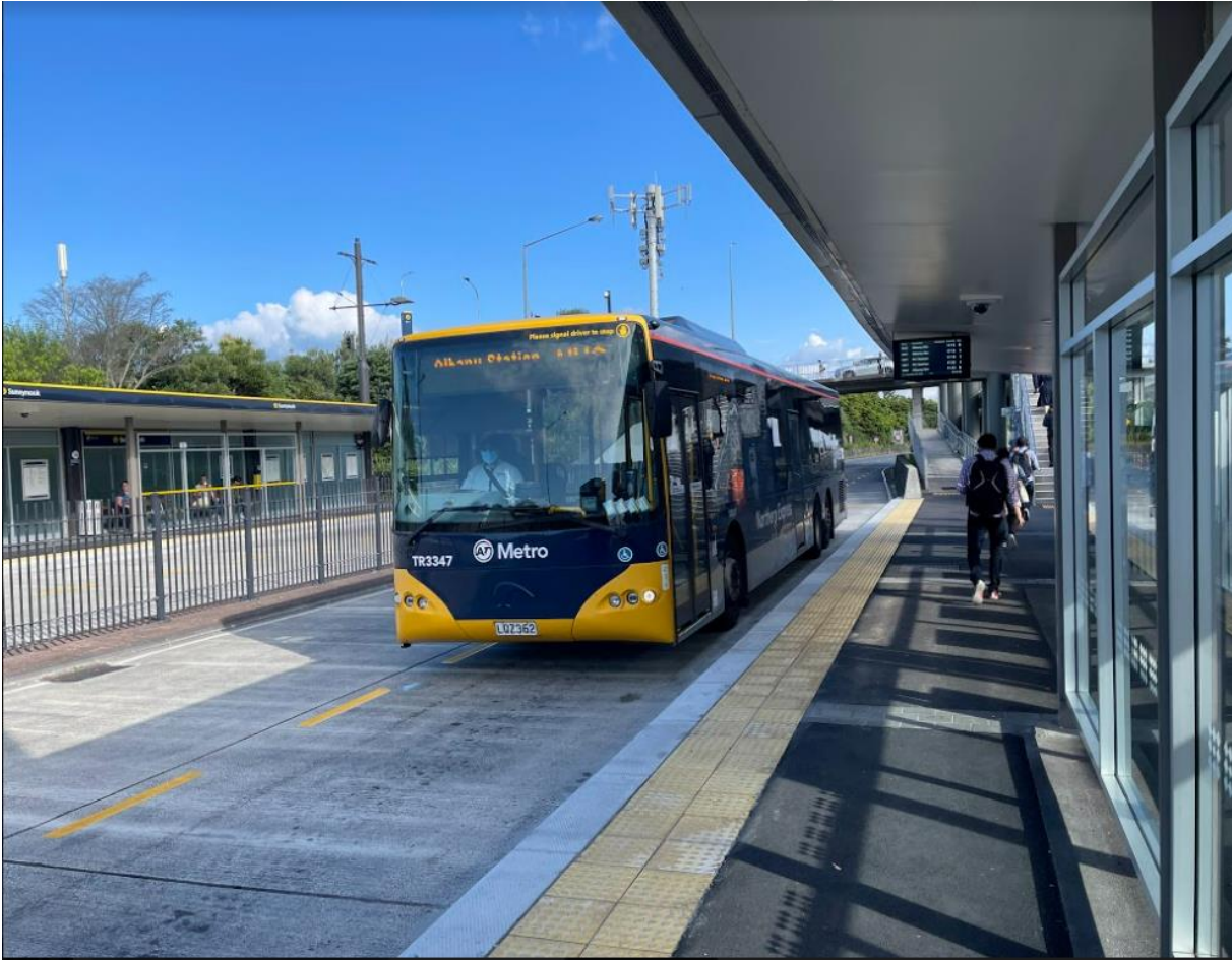
Figure 22: Sunnynook Bus Station. Source: Jacobs.
