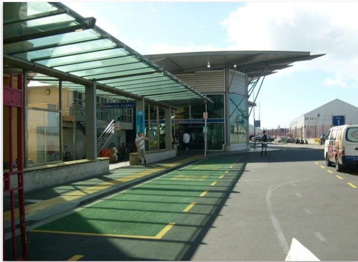
Figure 25: Bus box with coloured surface treatment, Auckland. Note: This stop does not appear to have adequate clearance. Source: Auckland Transport.
