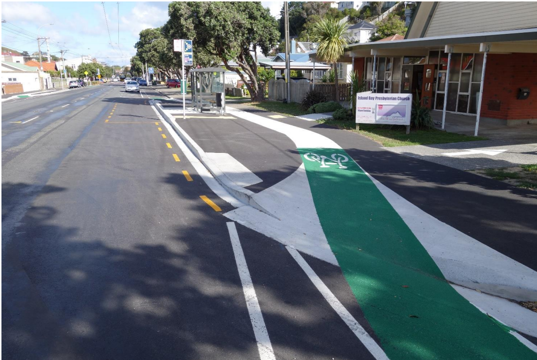
Figure 73: Full-width island bus stop. Note the lane markings and residual footpath widths are not optimal. Source: Simon Kennett.
