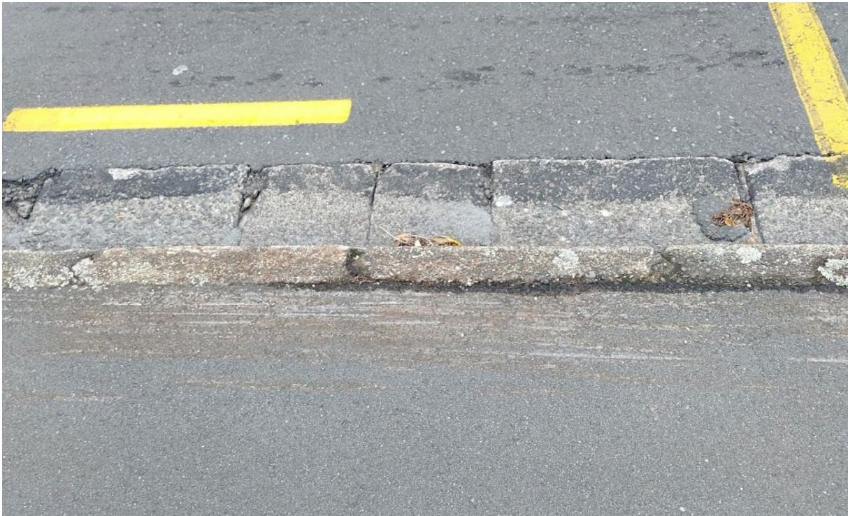
Figure 27: Damage to kerb and footpath from bus scraping associated with inadequate ground clearance (Source: Lorelei Schmitt)
