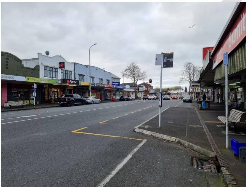
Figure 58: Full width bus boarder in Auckland. Source: Thomas Chu.
