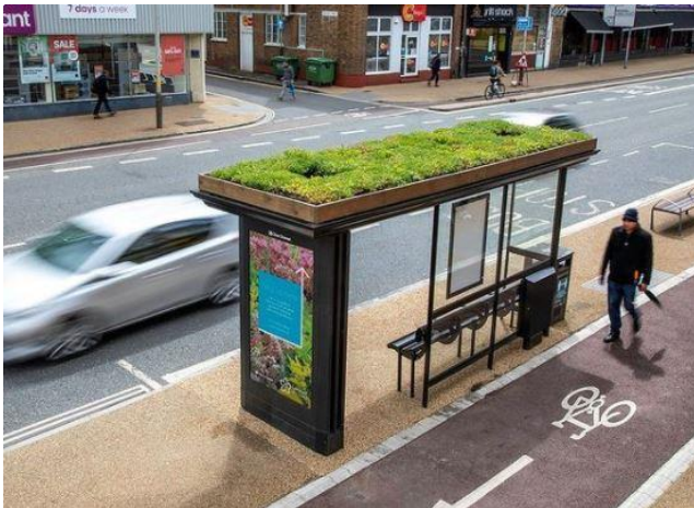
Figure 1: Green/living roof on a UK bus stop shelter. Source: Clear Channel UK.
