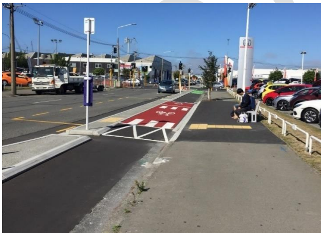
Figure 79: Nominal-width island bus stop (one-way cycleway), Christchurch. Note: Red under white crossing markings is not recommended. Source: Waka Kotahi.
