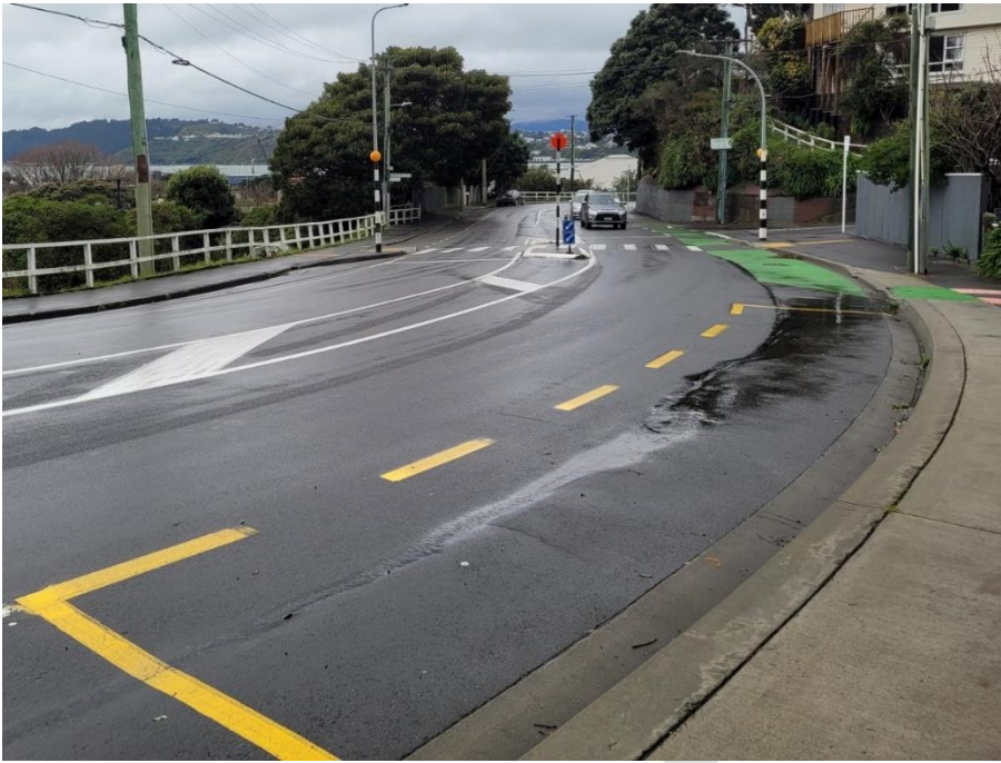
Figure 7: A zebra crossing located behind a bus stop encourages people to cross behind the bus (Source: Lorelei Schmitt)
