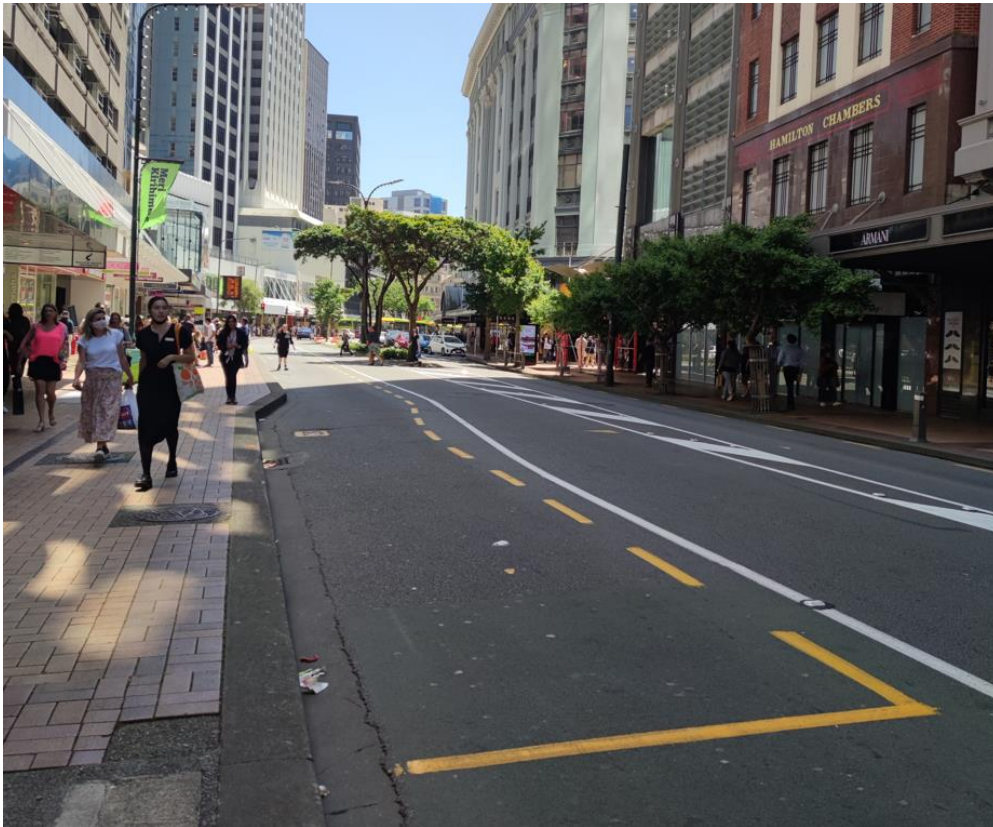
Figure 60: Half-width bus boarder in Lambton Quay, Wellington. Source: Joanne Tan.
