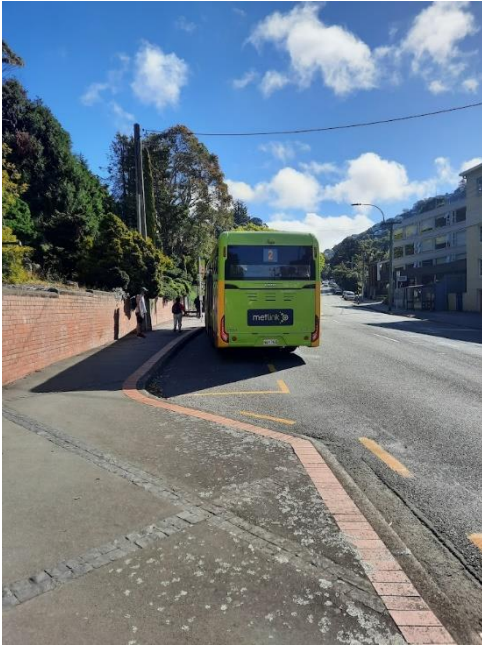
Figure 52: An indented bus bay with inadequate entry and exit angles resulting in bus drivers not pulling in closely to align with the kerb. Source: Lorelei Schmitt
