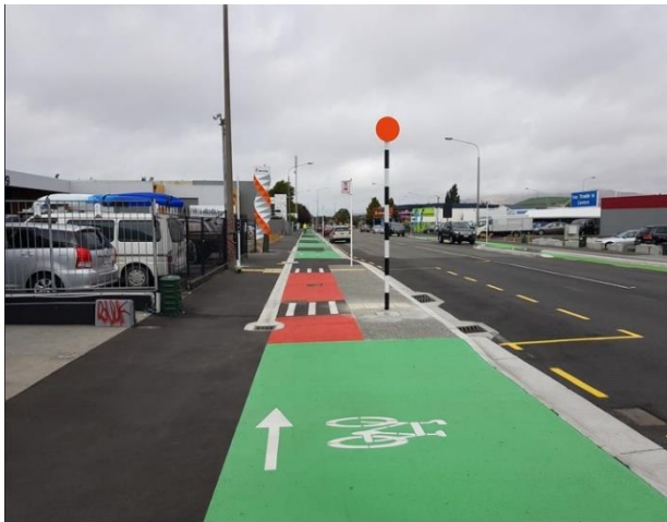
Figure 84: No red surface treatment under the white stripes (one-way cycleway). Note: Belisha beacons are not recommended. Source: Glen Koorey.
