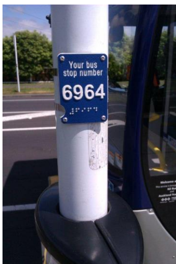
Figure 41: Signage showing bus stop number in digits and braille. Source: Flow Transportation Specialists.
