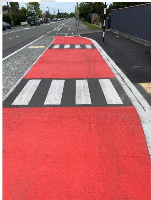
Figure 80: Nominal-width island bus stop (two-way cycleway), Christchurch. Note: the Belisha beacon is not recommended. Source: Simon Kennett.
