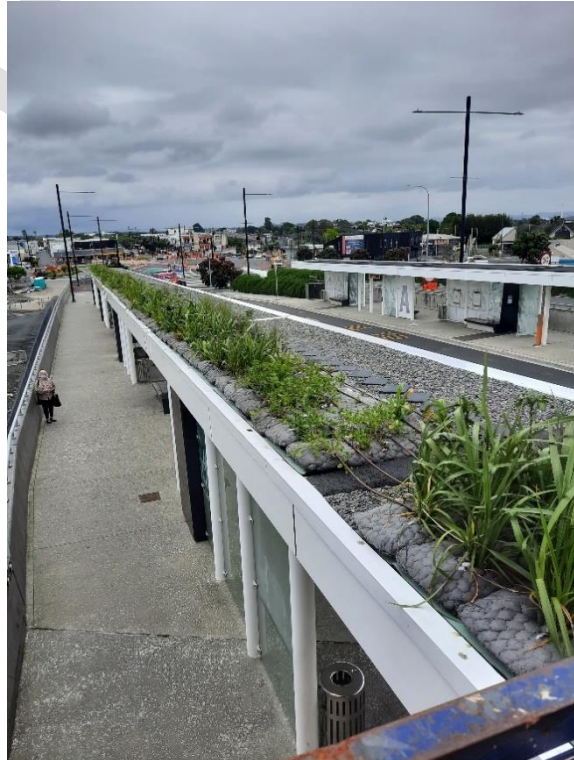
Figure 2: Green roof bus stop trials in Panmure, Auckland. Source: Cathy Bebelman, Auckland Transport.
