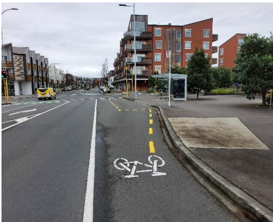
Figure 70: Cycle lane in a kerbside position, Auckland. Source: Flow Transportation Specialists.
