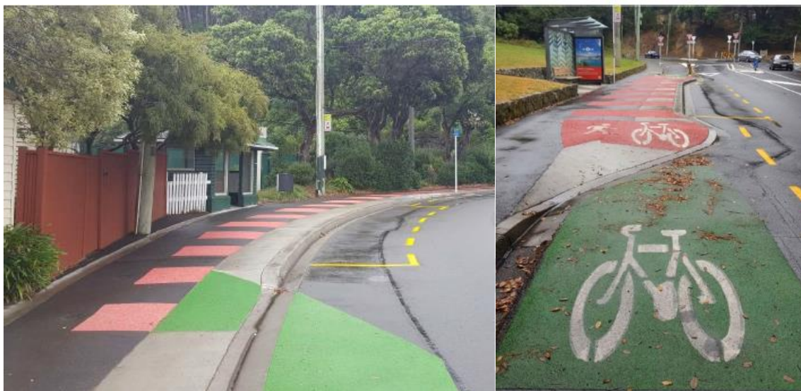
Figure 87: Shared space designs on Crawford Road, Wellington. Note: In the image on the left, cycle markings would indicate where people should bike. The pedestrian and cycling markings in the image on the right should be aligned vertically show it is a shared space and not 'lead' riders into the alighting zone. Source: Keren Love.
