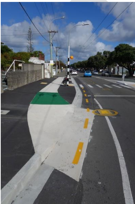
Figure 77: Narrow-width island bus stop. Source: Simon Kennett.
