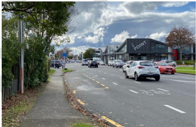
Figure 71: Cycle lane between a bus stop and a live traffic lane, Auckland. Source: Flow Transportation Specialists.
