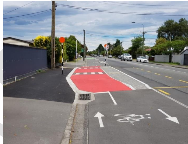
Figure 85: No red surface treatment under the white stripes (two-way cycleway). Note: Belisha beacons are not recommended. Source: Glen Koorey.
