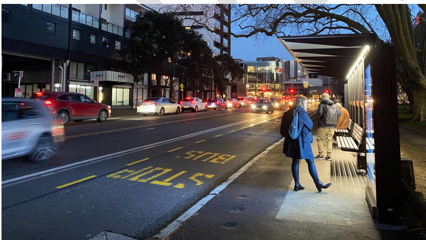
Figure 33: Bus stop shelter with lighting. Source: Elisa Hardijanto.
