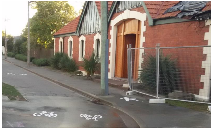
Figure 3: Pinch point on footpath at Matai Street site
