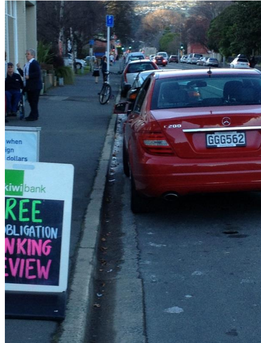
Figure 14: Flush transition from carriageway to channel
