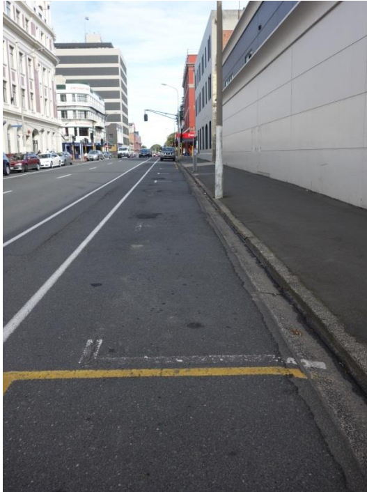
Figure 13: Lip at carriageway / channel boundary due to successive overlays
