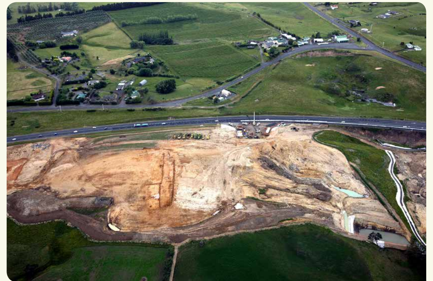
Project works for the Te Kauwhata Interchange
