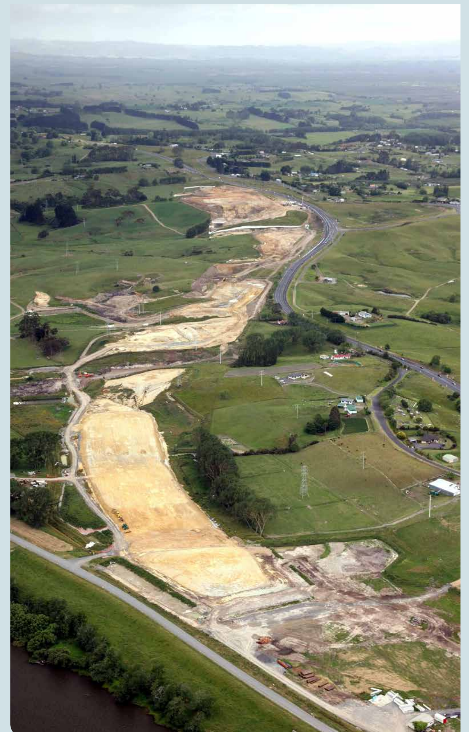
Top: Bridge piling at Rangiriri Bottom: Project earthworks
