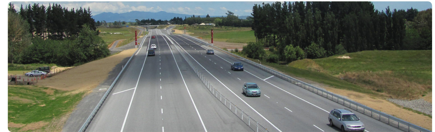
First day: The scene from the Lake Road bridge looking down to the new Waikato River bridge on the day the Ngaruawahia Expressway section opened to traffic, 16 December 2013.
