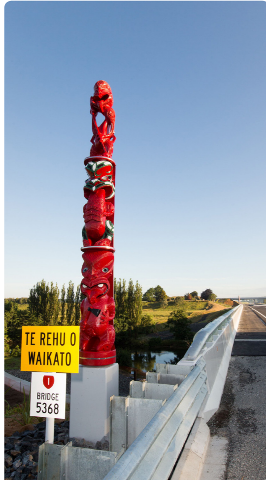
Standing tall: Two pou stand at each end of the new bridge.
