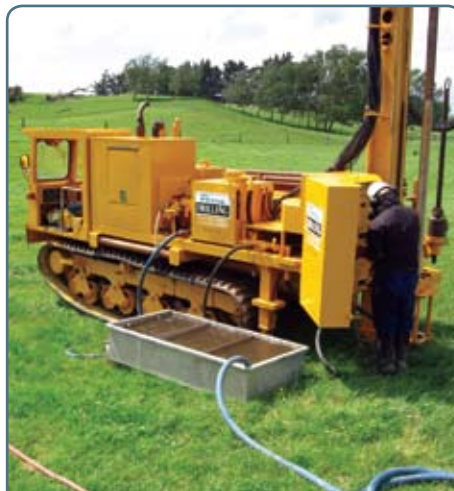
Geotechnical testing equipment being used on the Ngaruawahia Section
