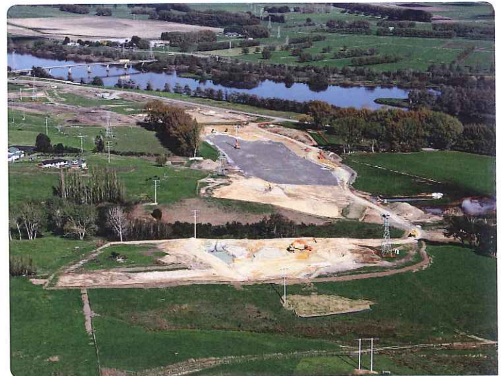
Aerial photo over the project area, looking south.
