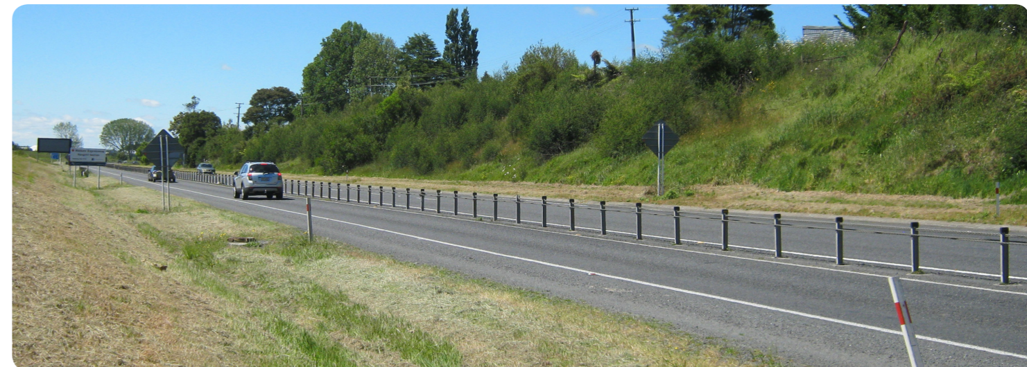
SH1 looking south
