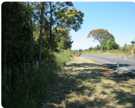
SH1 looking south
