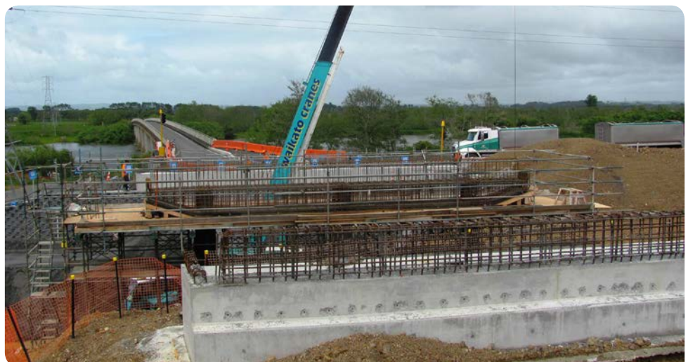
Work continues on the Rangiriri interchange
