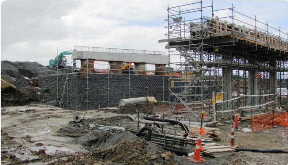
Te Kauwhata interchange is taking shape
